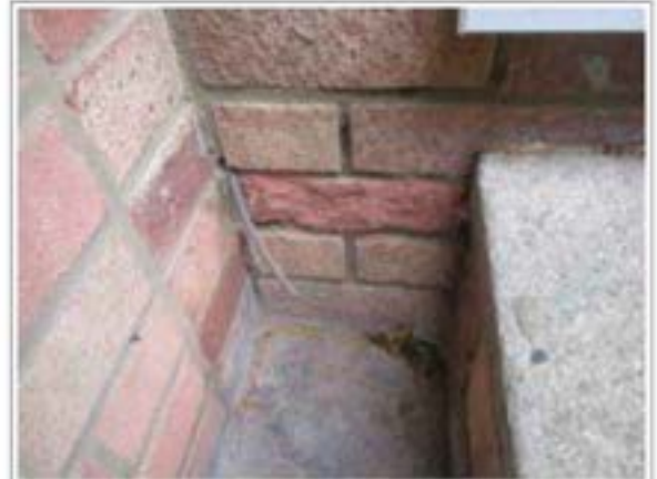
Eroded pointing
